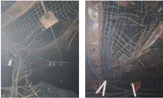
图 2 巷道冲击显现区域顶板变形破坏情况 Fig.2 Deformation and failure situation of roof in impact-prone area of roadway
