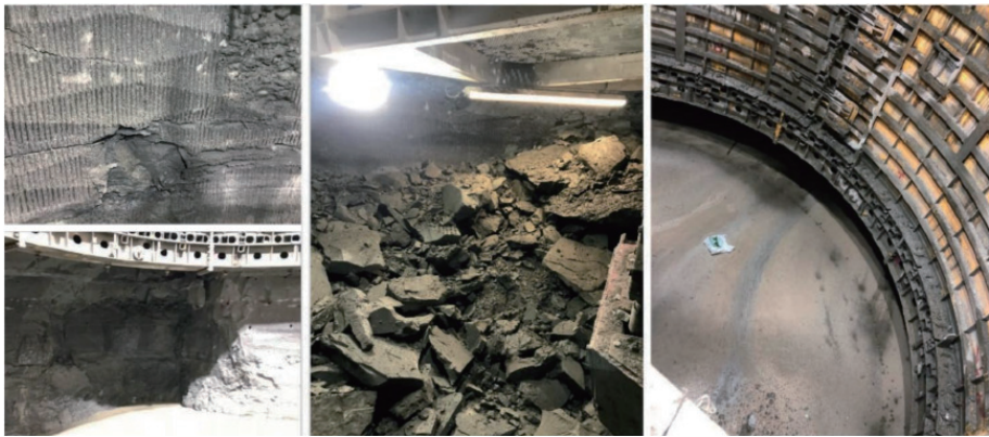
图 10 非冻结段井帮坍塌情况 Fig.10 Well wall collapse in non-frozen section
