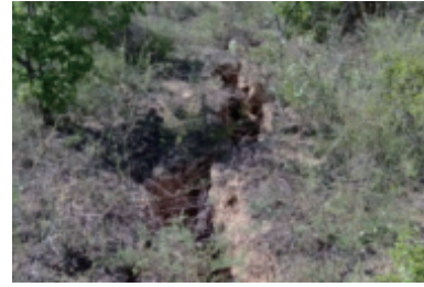
(a) 裂缝扩张
