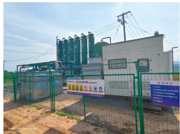
图 19 煤矿采空区分布式提纯系统 Fig.19 Distributed purification system for coal mined-out area
